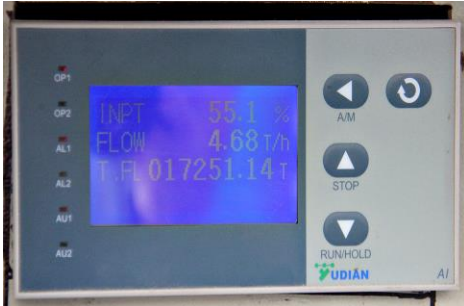
Steam Flow Meter Installed
